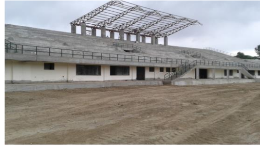
Shed sheets required to be installed on steel trusses
