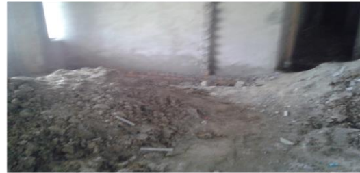
Bathrooms under construction
